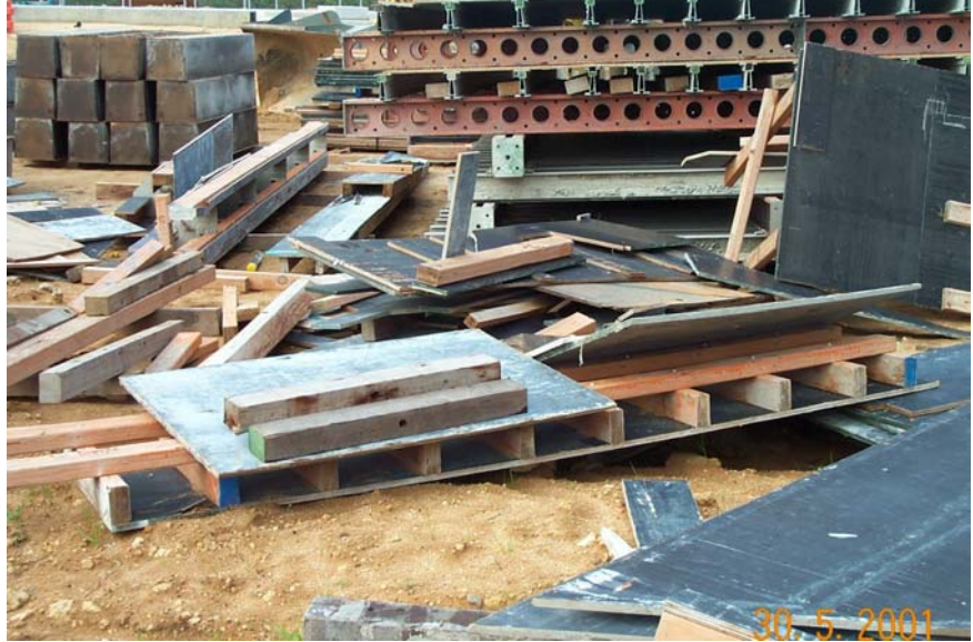
Construction waste collected and recycled on site at the Woodman Point Environmental Enhancement Project. In line with Western Australia's State Recycling Blueprint (1993), efforts were made by Halliburton KBR in concert with its Alliance Partners to minimise the generation, and maximise the recycling, of waste.
